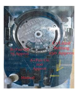
Once the fan and limit controller has been set it is time to start a fire to burn off any residue left over from manufacturing. This needs to be done before the duct work is connected so the fumes do not enter any enclosed space.
