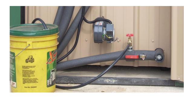
Plumb a garden hose bib (spigot), and a gate valve into the return line of each heat loop. To check the gpm flowing thru each loop.
